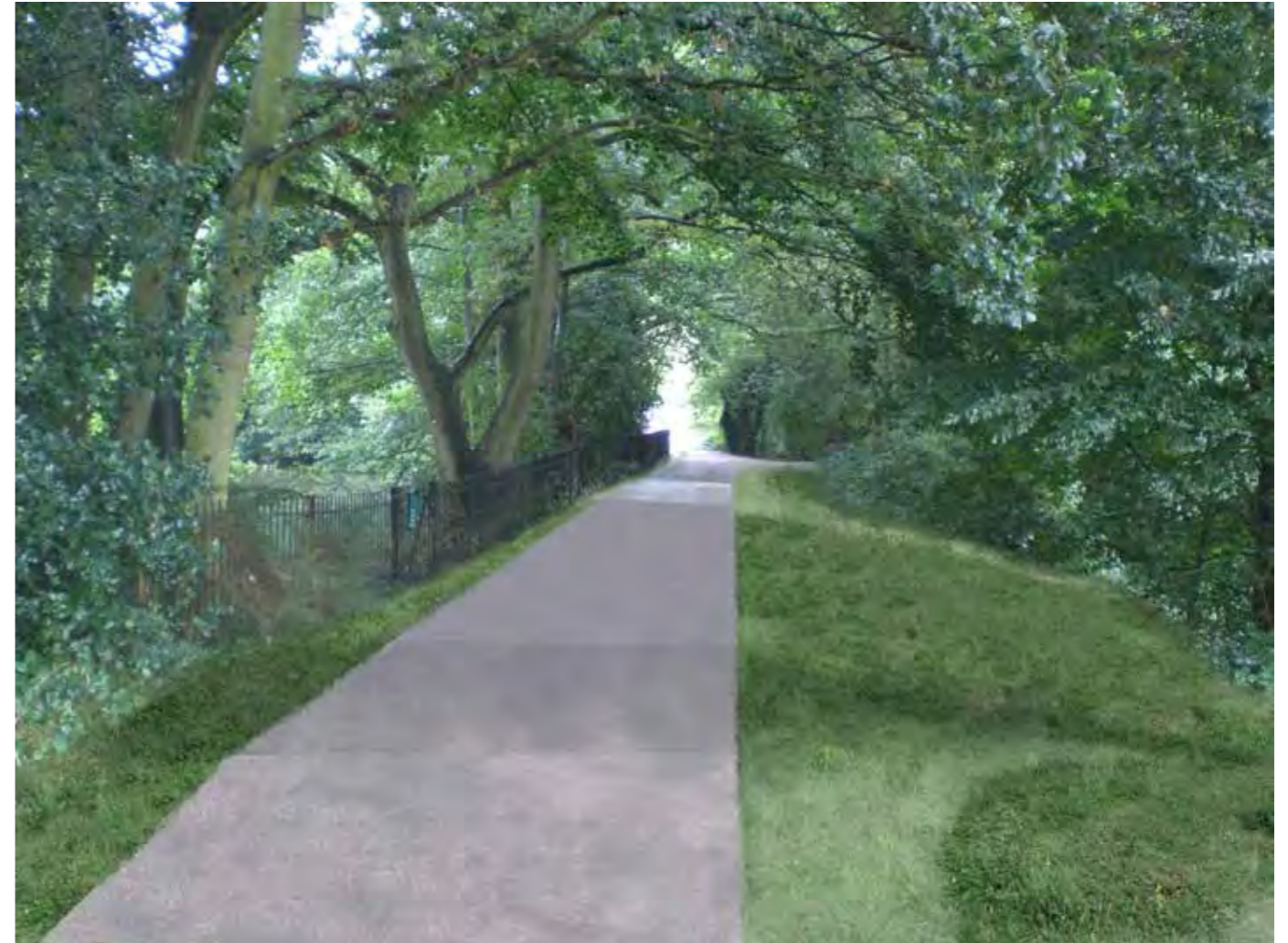
View Point 12 – View to north east of spillway along dam from south west of Stock Pond
