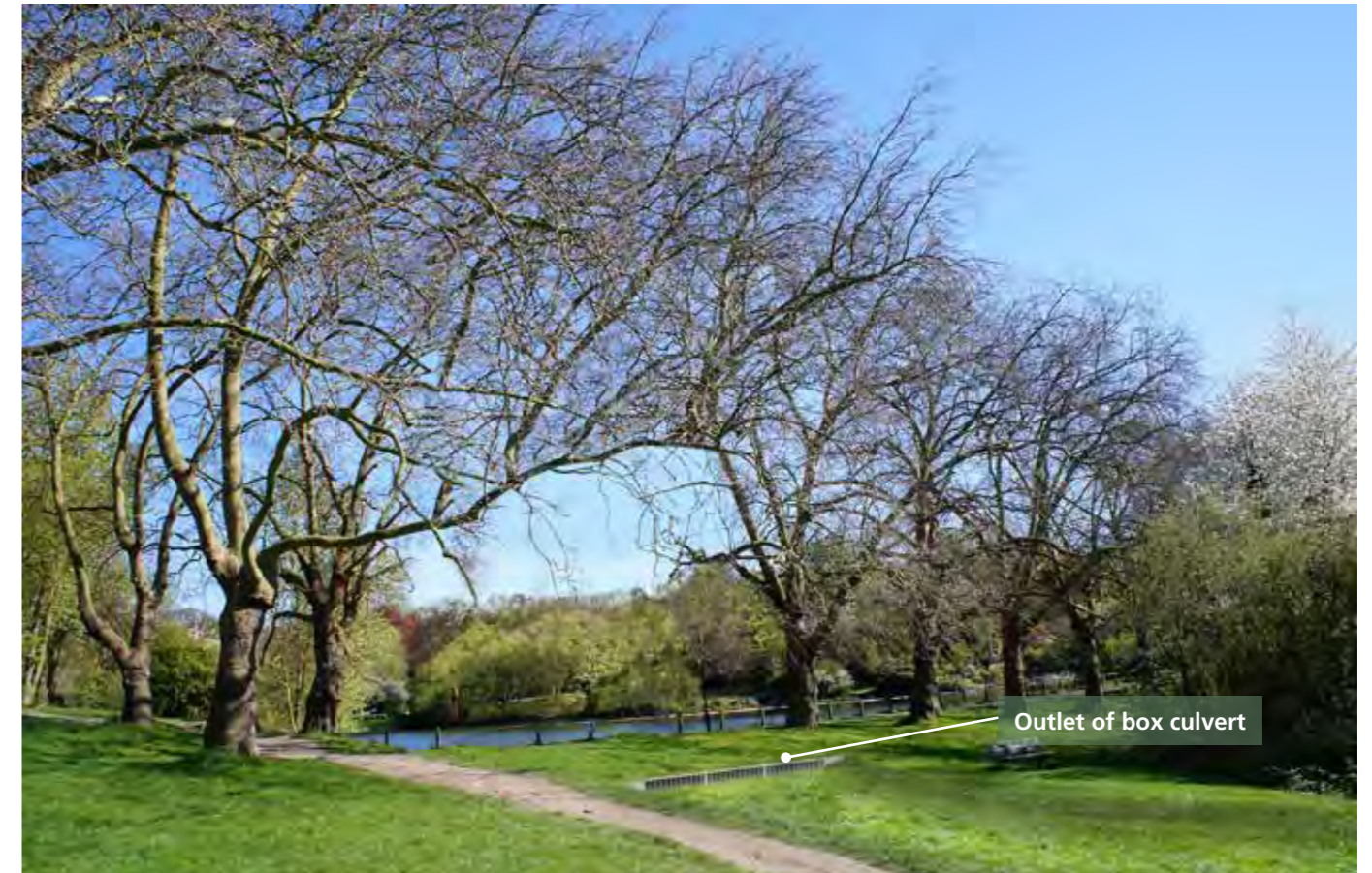
View Point 3 – North across Hampstead No. 2 Pond Box Culvert Spillway – 2 Plane Trees Lost, 3 x (300 x 3000mm) culverts (option M)
